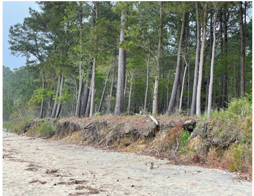
Existing Erosion at Park Shoreline. Photo by Mary Terry
